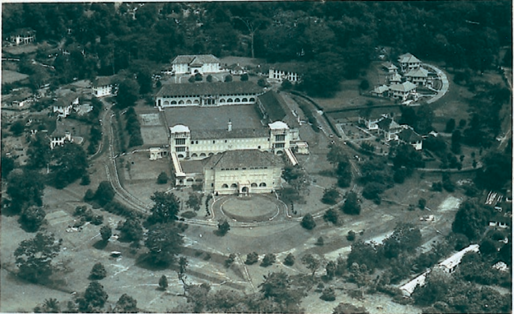
Aerial View of the Bukit Timah Campus of the University of Malaya.
