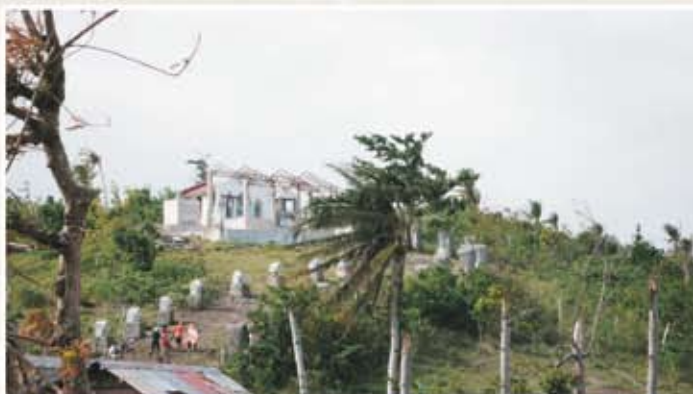
Uphill walk along Stations of the Cross path to ruined chapel
